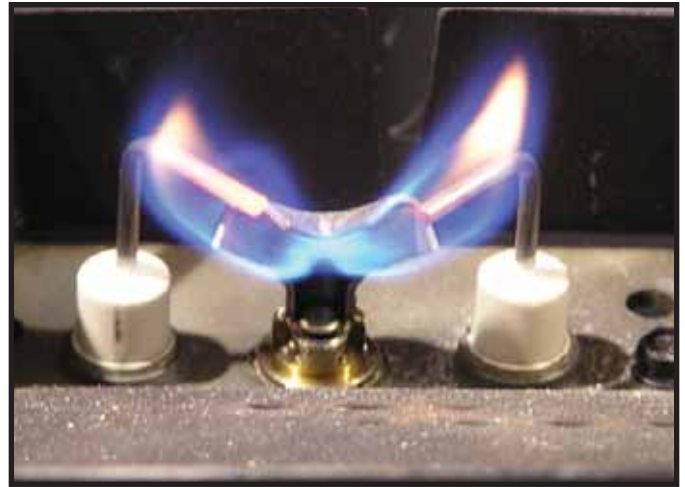
Figure 3.1 IPI Pilot Flame Patterns
